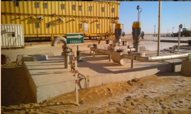
Open drain pit and pumps on the artificial island
